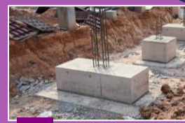
Pad Used with poor soil to create a strong, yet shallow foundation
