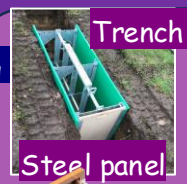
Trench support Steel panel Trench box
