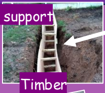
Timber Interlocking sheet pile
